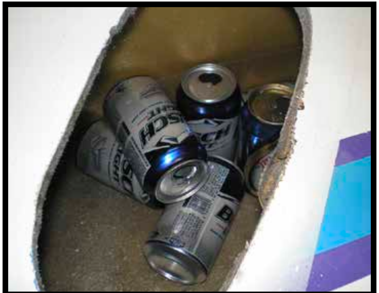
Repairs on Y-2762 revealed archeological proof that the hull was, indeed, built by Chet.
